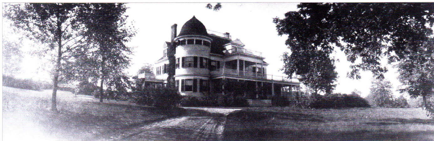
Tarry-A-Bit soon after construction.
